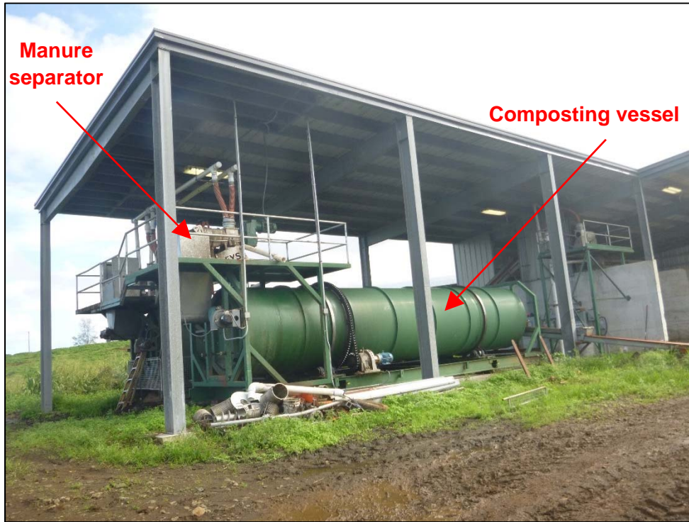
Photograph 17. View of the Facility's manure composting building which included two manure separator units, and two composting digester vessels. Photo by A. D'Angelo; 12/14/16.
