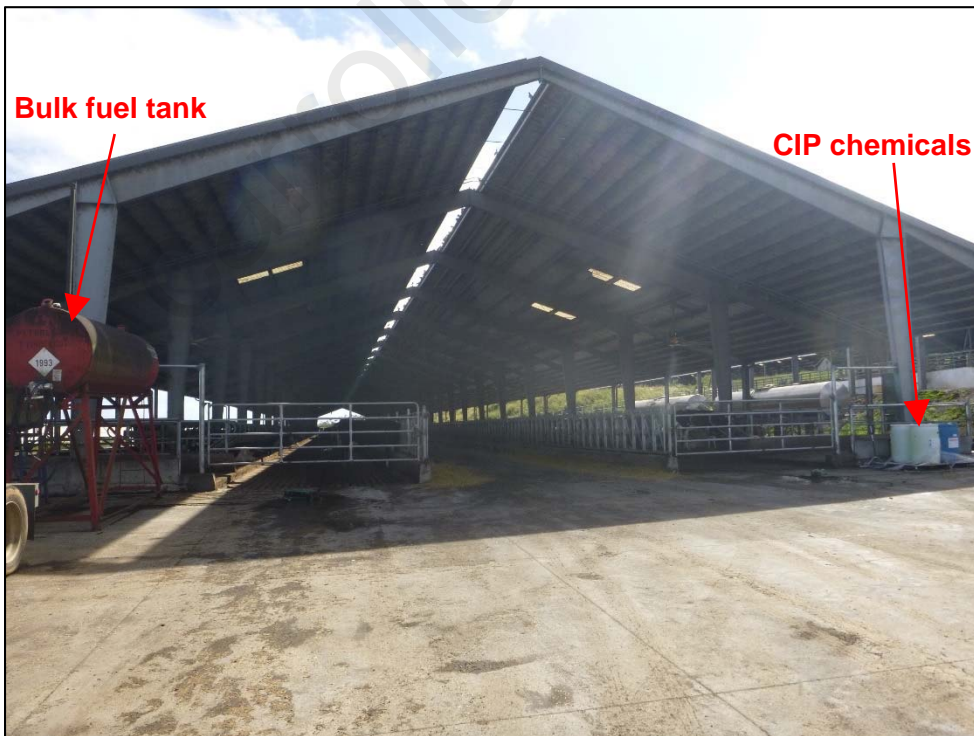
Photograph 4. View of the Facility's newly constructed lower 1,000-cow freestall barn. Note the bulk fuel tank and CIP chemicals. Photo by A. D'Angelo; 12/14/16.
