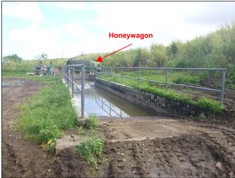
Photograph 15. View of the Facility's manure composting building collection pit. Waste streams from the freestall barns, calf barn, and milking barn gravity flow into this collection pit. Note the honeywagon stored behind the collection pit. Photo by A. D'Angelo; 12/14/16.
