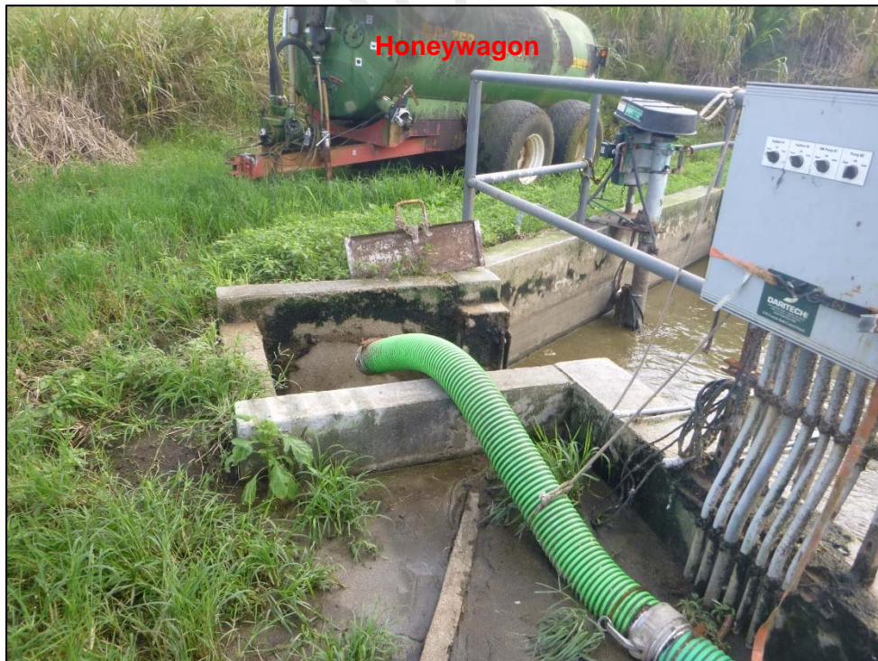
Photograph 20. View of the manure composting building collection pit overflow point. Overflow flows into the manure separation cells shown in Photographs 22 and 23. Note the honeywagon. Photo by A. D'Angelo; 12/14/16.
