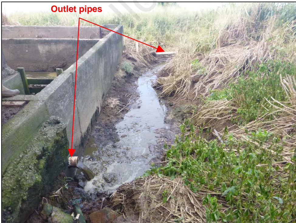
Photograph 24. View of the two pipes that drain separated liquid from the manure solids separation cells. Liquid from the cells surface flows, via an earthen conveyance channel, into the northwest side of the upper lagoon. Photo by A. D'Angelo; 12/14/16.
