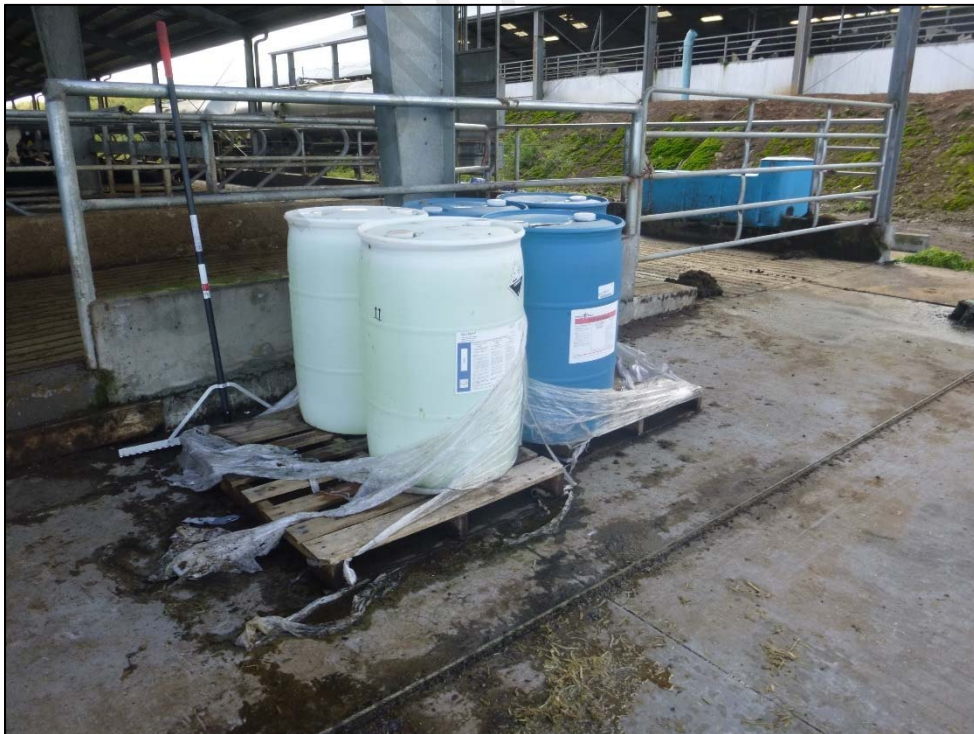
Photograph 10. View of two 55-gallon drums of acid and two 55-gallon drums of caustic detergent used in the milking barn CIP system. The drums were stored outside, without overhead coverage or containment, and in close proximity to each other. Photo by A. D'Angelo; 12/14/16.
