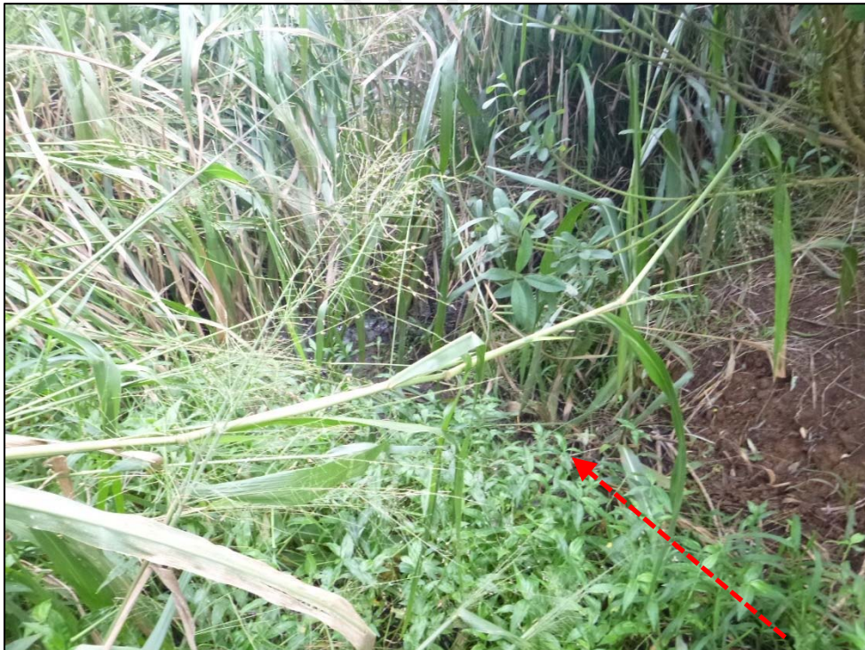
Photograph 36. The channel downgradient of the lower lagoon overflow spillway was heavily vegetated; however, I observed clear channelization and a flow pathway toward Kaohaoha Gulch. Photo by A. D'Angelo; 12/14/16.
