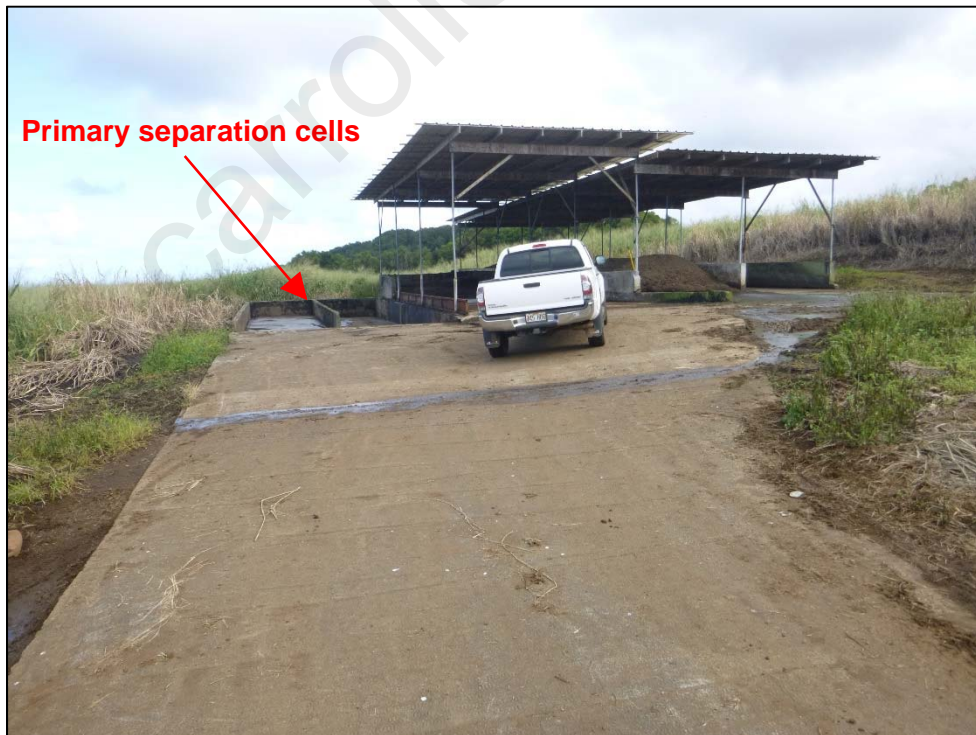
Photograph 22. View, facing east, of the Facility's manure solids separation cells located adjacent to the upper lagoon (refer to Figure 2). The uncovered cells on the left serve as the primary cells and liquid waste discharge points. Photo by A. D'Angelo; 12/14/16.
