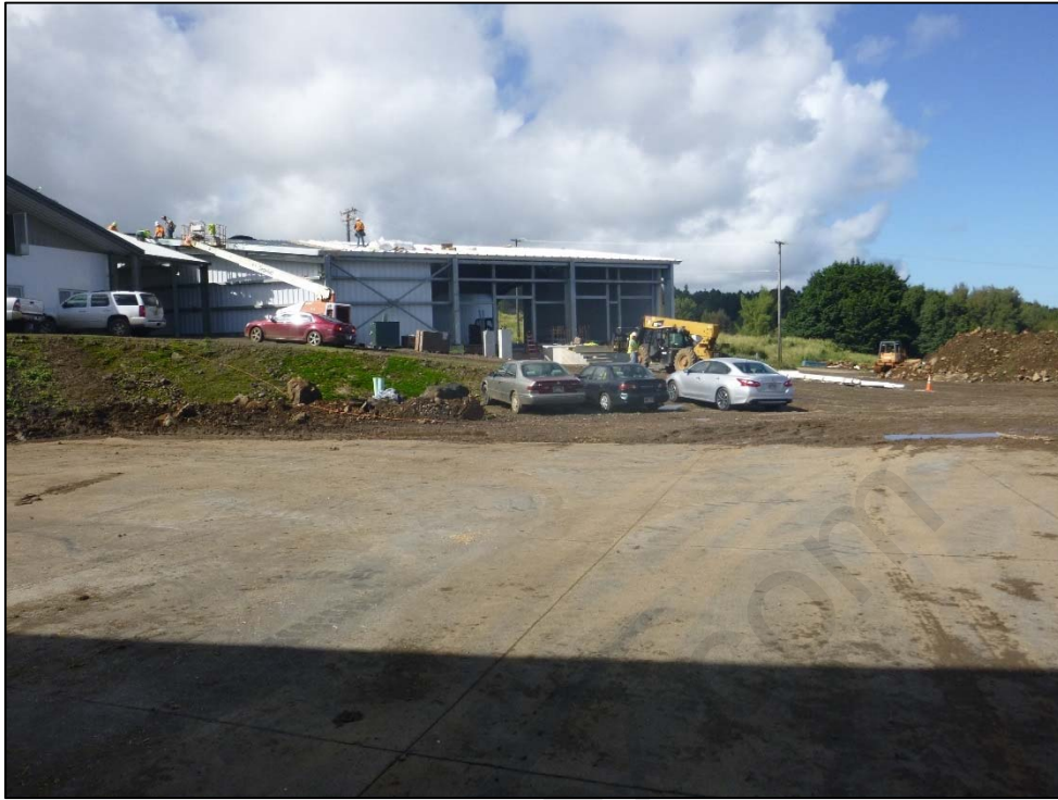
Photograph 3. View of the Facility's new building that was under construction at the time of the inspection. Photo by A. D'Angelo; 12/14/16.
